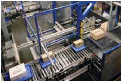
Above: Our distribution centre in Terrebonne, Québec uses state-of-the-art technology to improve efficiency and service to our stores.
